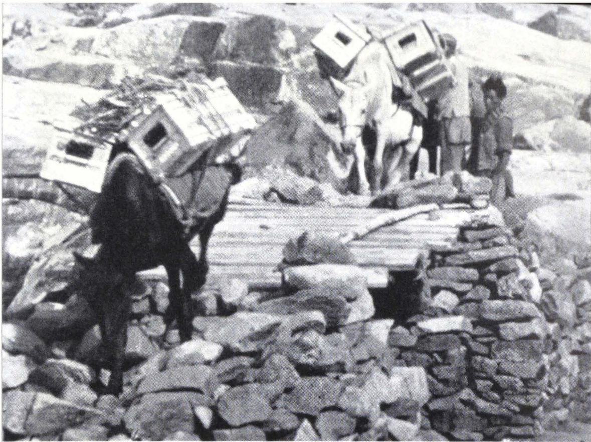
Crossing a Seasonal Bridge Bridges of this type are rebuilt every spring.
